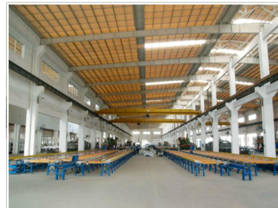
Extrusion production line
